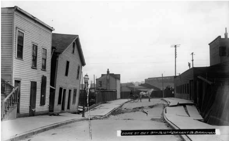
"Dore Street, Earthquake, 1906," site of the fabled Dore Alley Street Fair, between 9 th and 10 th streets, SoMa. Gay culture South of Market was built on quivering fill. In 1989, the Loma Prieta earthquake destroyed the Drummer office, and, in effect, the Drummer business whose coup de grace came from the Internet.
